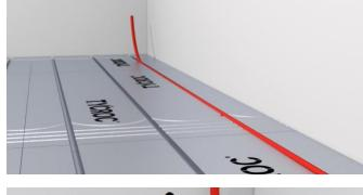
Push the heating pipe into the grooves using your foot or hand, ensuring it is properly seated. Confirm that the pipe extends to the connection point and leave an additional 1 meter of extra length for adjustments.
