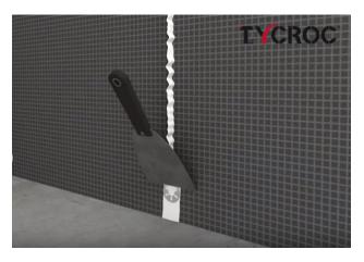
The gaps between building boards and corners should be covered with adhesive sealant, and also fastening washers should be covered with the help of a spittle.
