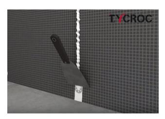
The gaps between building boards and corners should be covered with adhesive sealant, and also fastening dowels should be covered with Tycroc Premium FIX adhesive. Direct water contacted corners, cover additionally with waterproofing tape and —membrane.
